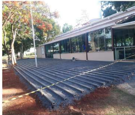
Attention: put crushed stone or stone powder between the structure lines.
